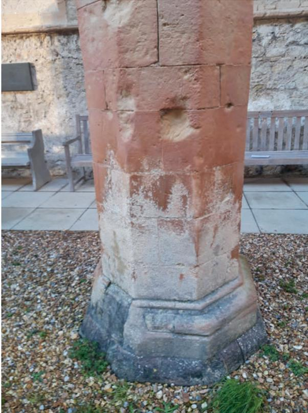
*Figure 3. Combined bomb blast, fire, and salt weathering damage on a pillar of the Royal Garrison Church, Portsmouth, UK. Photograph by the author.*
