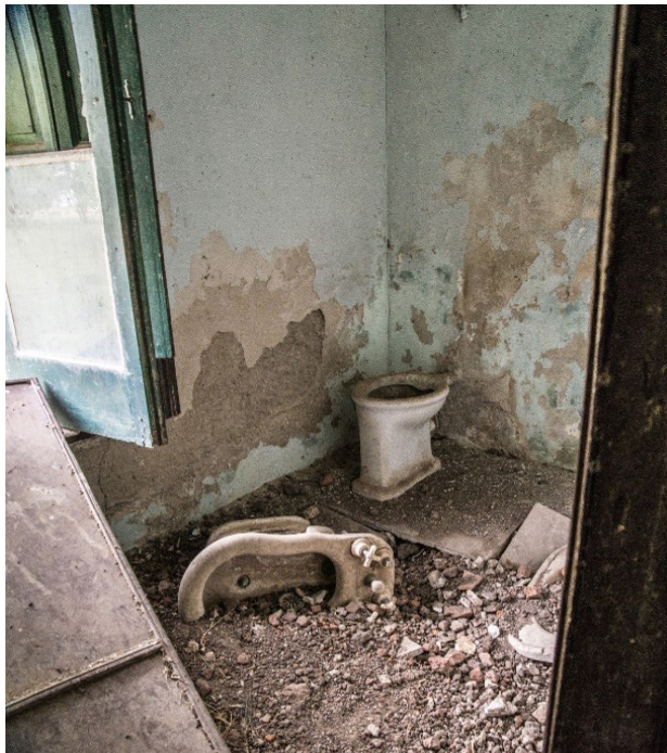
Photo 9. Old abandoned estancia house.
