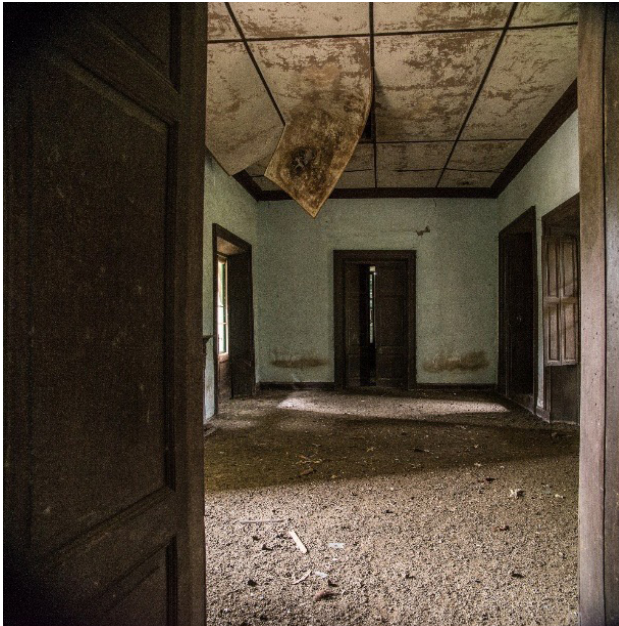
Photo 8. Old abandoned estancia house.
