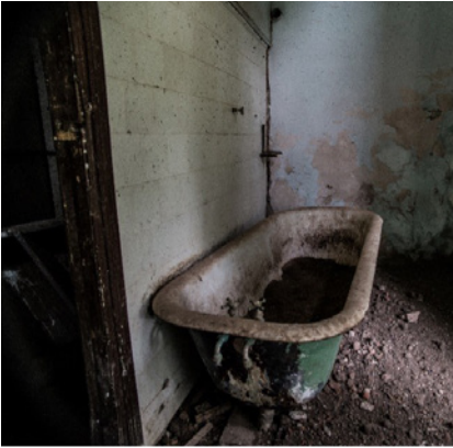
Photo 10. Old abandoned estancia house.
